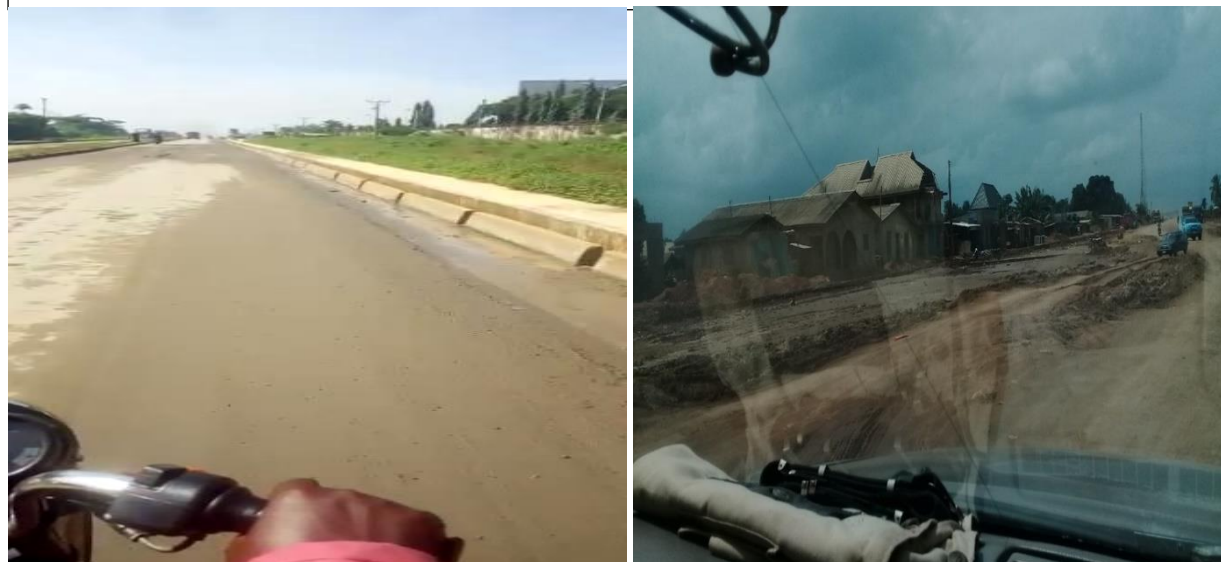
Fig. 5.2.3: Lusada-Igbesa Road Condition progress in Dec.2020 & initial condition in July 2019 when construction started.
