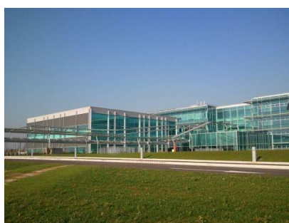
Figure n.20: Former Microsoft Italia building in Peschiera Borromeo (MI)
