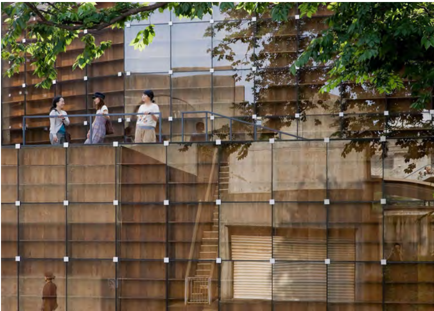
Figura 268 - Terraço exterior. © Iwan Baan
