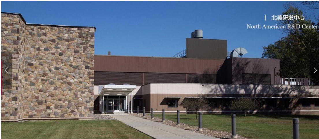
Figure 4.23 Oriental Yuhong Company North America R&D Center
