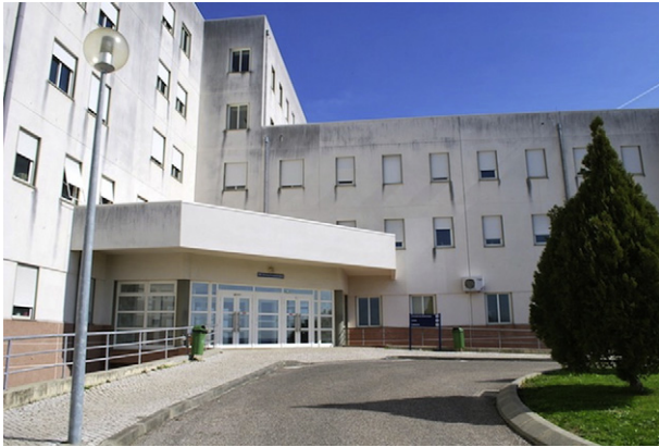
Fig. 7. External space of the new G hospital.
