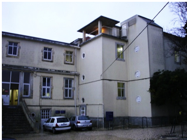
Fig. 4. External space of the old O hospital.
