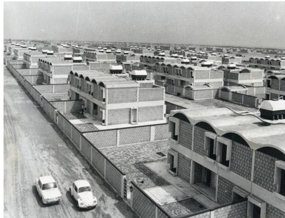
Al Rikka City Prefab low income 2330 Kuwait Engineering Bureau + Jafar Tukan 1971-76
