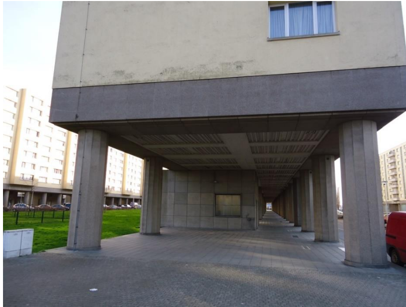
Figure 16: View between the pillars. The floor is paved with concrete tiles, while the ceiling between the bunks of 1,2 metre high, are equipped with ribbed concrete slabs. (photo: Els De Vos, 2015)
