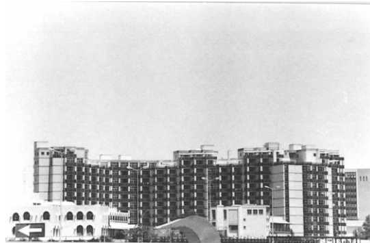
Fig. 23 United Center Housing Complex , Georges Candilis project and photo 1975
