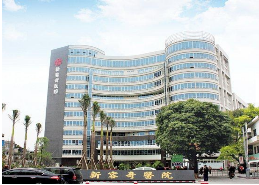
Figure 5-10 New Outpatient Building of R Hospital
