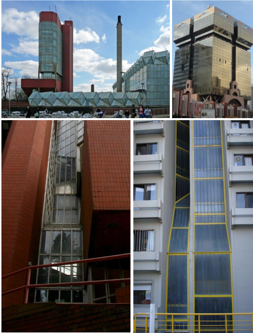
34. Leicester Engineering Building, James Stirling, 1959-63 [Fonte: http://www.studyblue.com/notes/note/n/history-exam-3-building-ids/deck/6312321 ]
