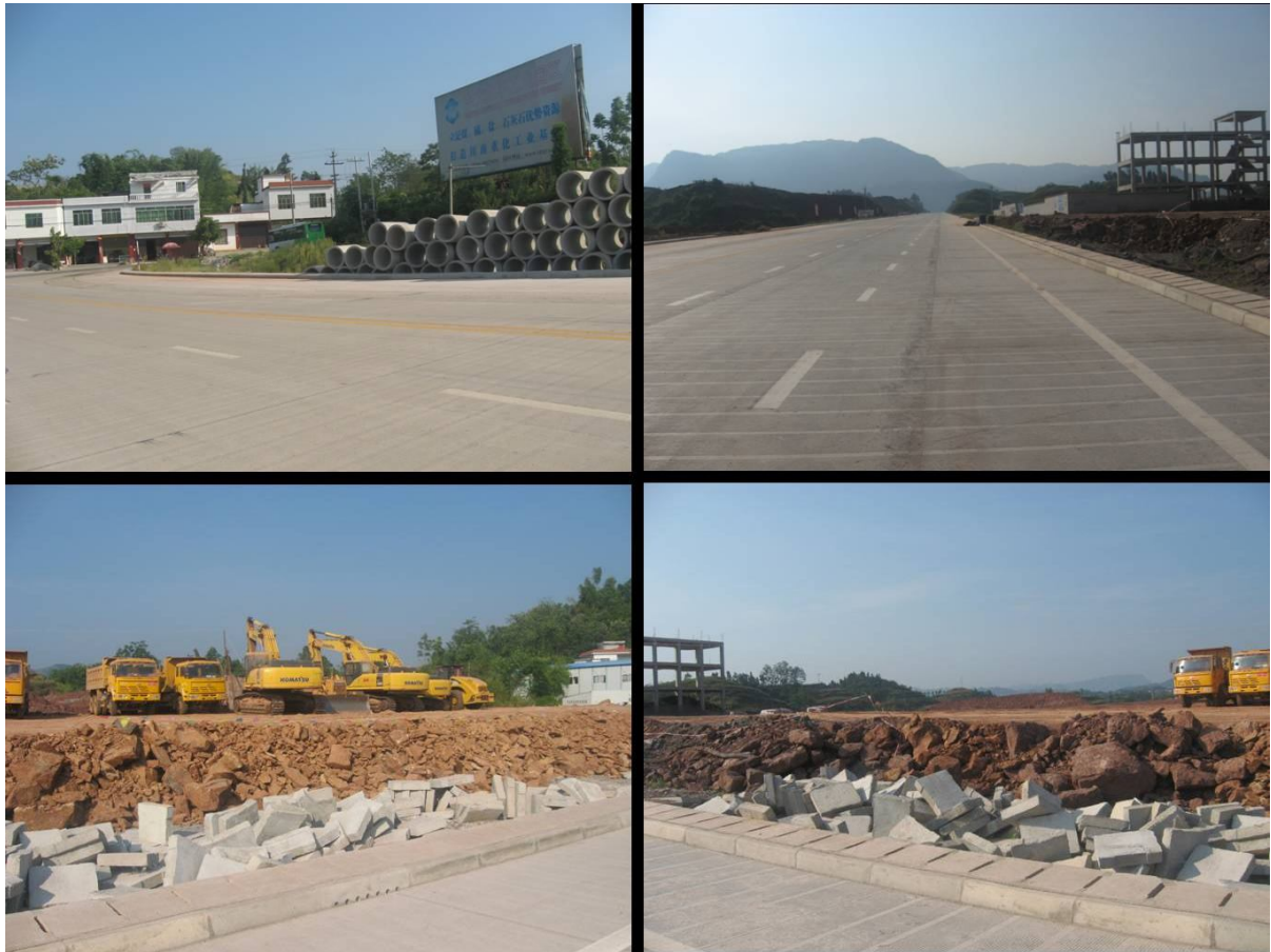
Photo 1-4: High Street Construction Site
