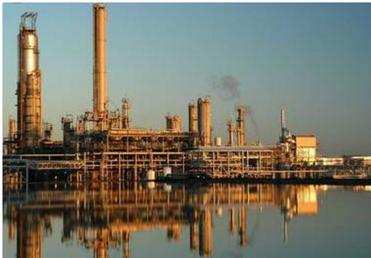
Figure 4: Galp Energy's Refinery in Sines Source: Galp Energy
