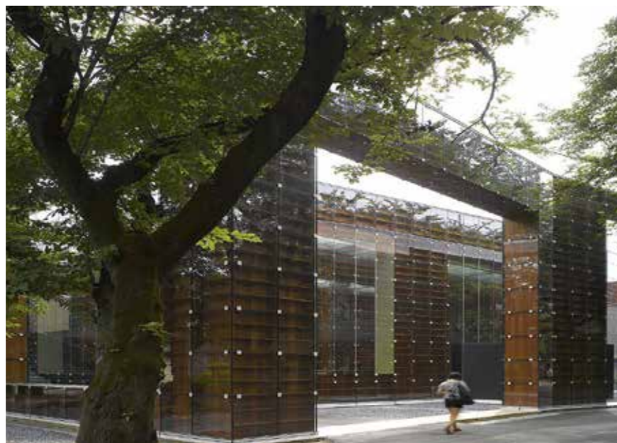
Figura 269 - Parede exterior. © Edmund Summer
