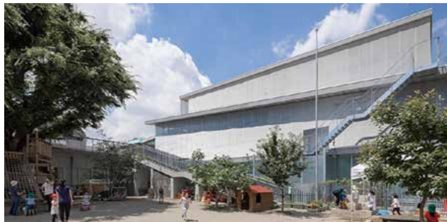
Figura 386 - Fachada sul. © Vincent Hecht
