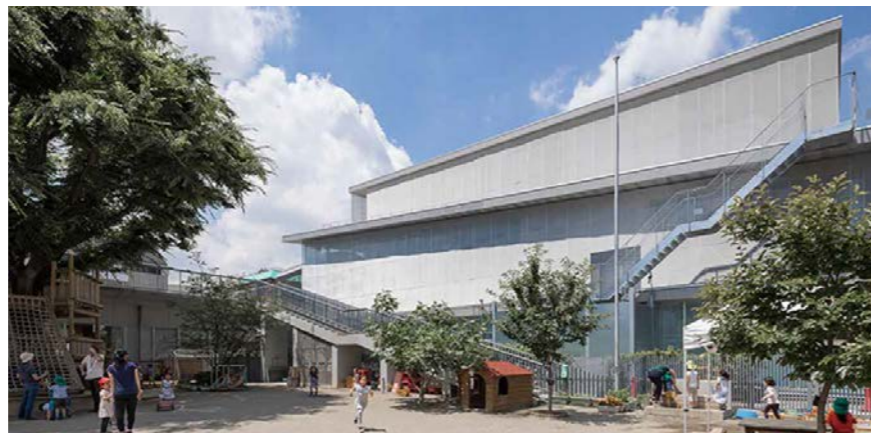
Figura 386 - Fachada sul. © Vincent Hecht
