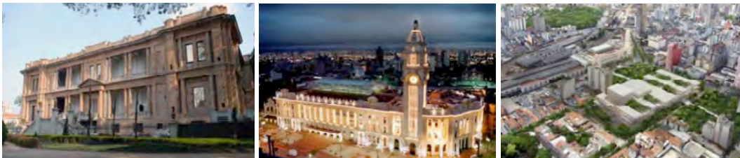
6. Pinacoteca do Estado | Sala São Paulo | Center for Music and Dance Source: Municipality of Sao Paulo
