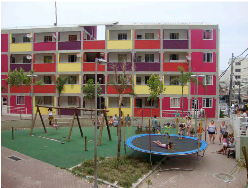
Figures 4 and 5: New constructions in Rocinha, built to relocate dwellers of one of the main local streets, that was enlarged in order to allow the circulation of vehicles.
