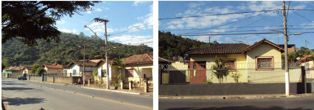
Figures 39/40. Larger type (engineers's houses). (Source: Jaqueline Duarte, 2011).
