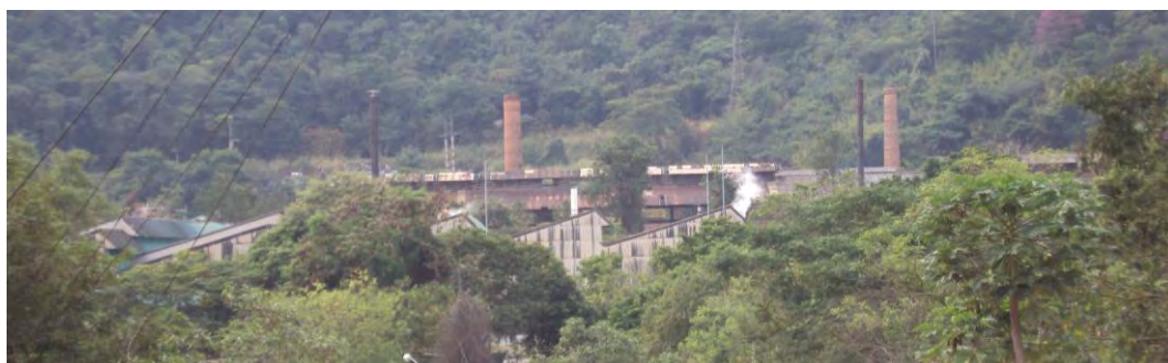
Figure 42. Sheds and smoke-stack inserted among the vegetation, characterizing the huge equipments that compose this urban tissue. (Source: Jaqueline Santos, 2011).
