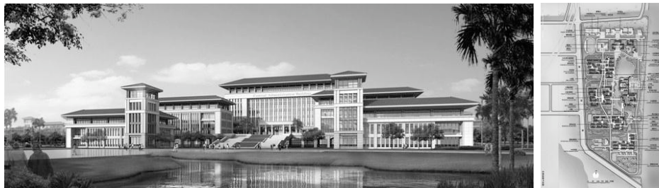
Figure 05. Layout aspect of a building and plan of the Macau University Campus at Hengqin Island.
