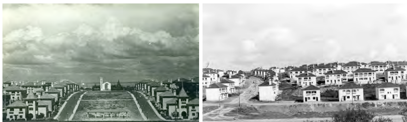
Figure 7: Encarnação Neighbourhood construction (Portugal 1951; - c.1940)
