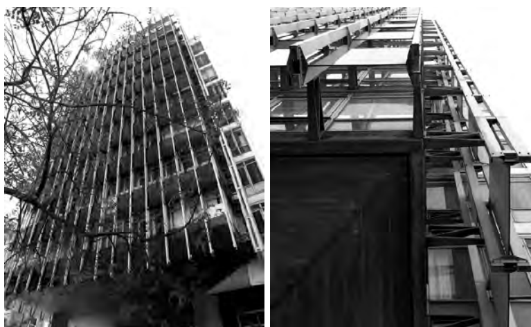
Fig. 8 - Detail of the façade and its components. Source: photos by Mariana Porto Ferreira, 2013
