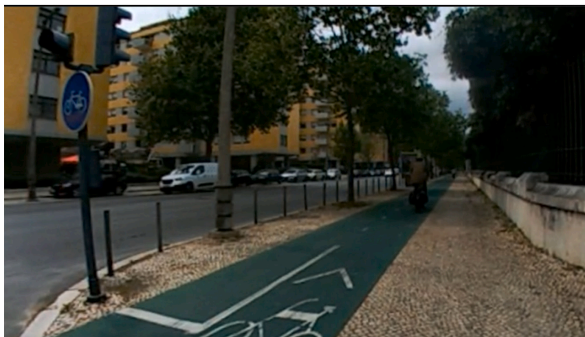
Fig. 13. Cycling indication as a sign and floor painted (Avenida do Brasil).
