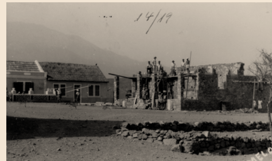
Fig. 17. Porto Novo (?), Santo Antão Island, Cape Verde, 1948. Being “modern or progressive” in Cape Verde often meant simulating contemporary design by using local techniques and materials. However, the use of basalt stone, which was abundant in the region, determined the design applied. Source: No Arquipélago da Sede e da Fome , Higher Inspector of Colonial Administration António de Almeida, AHU, A2.01.02.009/0045.
