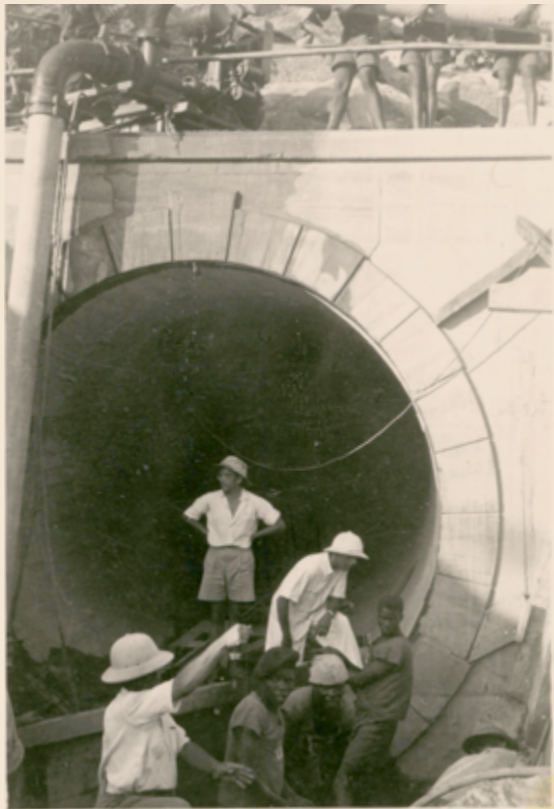
Fig. 1. Mabubas Hydroelectric Dam/Power Station, Angola, 1948. Concreting of the threshold. Inspection report of the Mabubas Dam (formerly known as President Craveiro Lopes Dam), by the engineer António Pinto Coelho*. There were three 8-hour working shifts. In October, the month covered by the report, it was also noted that "despite the intensive work regime", the "state of health" of the workers was "more than satisfactory," with only 1.7% registered as unhealthy. The search for new sources of energy, in particular hydroelectric power, would be one of the key programmes to promote the development narrative of the Estado Novo regime. This dam was one of the first large-scale modern achievements of its kind in Angola. Source: Aproveitamento Hidro-elétrico das Mabubas, Fiscalização das obras: Relatórios do engenheiro chefe , AHU, OP3010.
