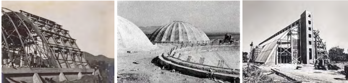
Figure 3. ( left ) The ‘ctesiphon’ shell constructed by its inventor Irish engineer, James Waller, circa 1940s (Hawkins, Will, et al. 2016); ( center ) Cast-concrete grain containers circa 1950s (Georgiou, Costas. 2018); ( right ) Carob warehouse in Limassol built in 1961 by the Tekton Technical office of Foivos Polydorides and Andreas Papadopoulos. (ereos, Stefanos, Aimilios Michael, and Irene Hadjisavvas-Adam, 2009).
