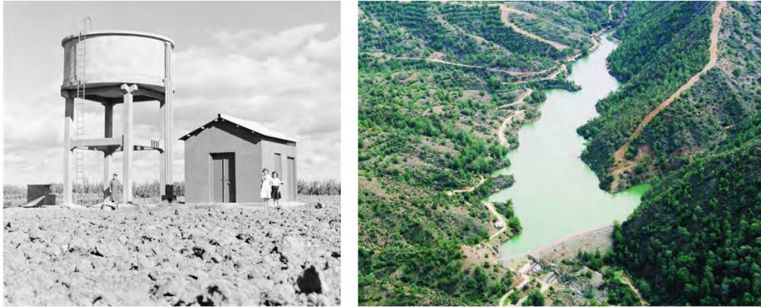
Figure 1. (left) Typical village pump-house and elevated irrigation tank used for the Greater Nicosia Water Supply Scheme. Source: Press and Information Office of the Republic of Cyprus, “Water Supply and Irrigation 1950s” folder, 28A-0049-0002, circa 1950s; (right) Argaka Dam built in 1964, commissioned to Howard Humphreys & Sons, the same company which designed the Greater Nicosia Water Supply Scheme. Source: Water Development Department, 2009. Dams of Cyprus, Nicosia.
