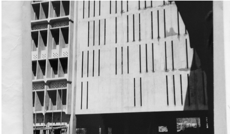
Figure 14. Pre-cast Lattice Work window detailing and slits for light and view out from pedestrian passageways (Archivio Ponti, Studio Salvatore Licitra).
