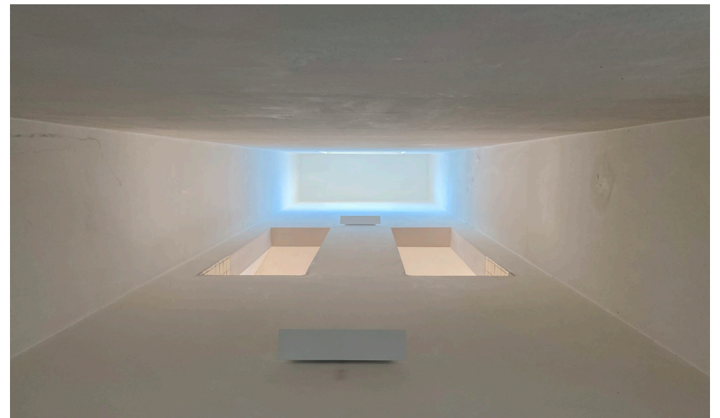
31. Lightwell in the north façade that illuminates the space behind the altar, with two openings, and below this, the mortuary chapel space.
