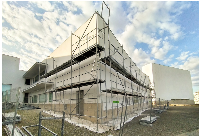
55. 56. Replacement of exterior wall cladding materials for the church and parish centre.
