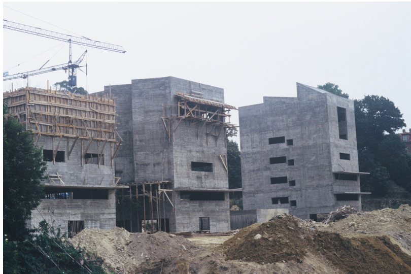
24. Construction of the concrete structure.
