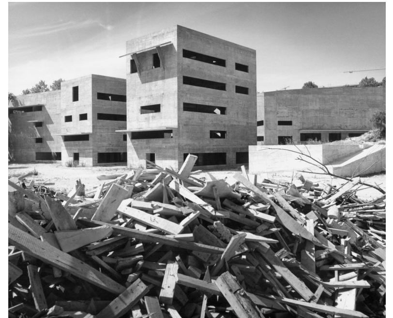
25. 26. Concrete structure during construction, 1990.
