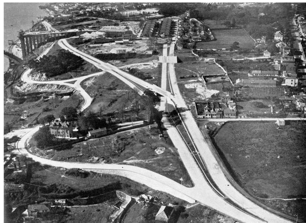
06. Quinta da Póvoa during the construction of the Arrábida bridge
