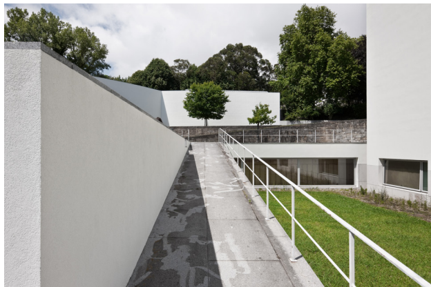
08. Ramp between the towers.
