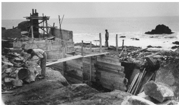
20. Laying of the foundations.
