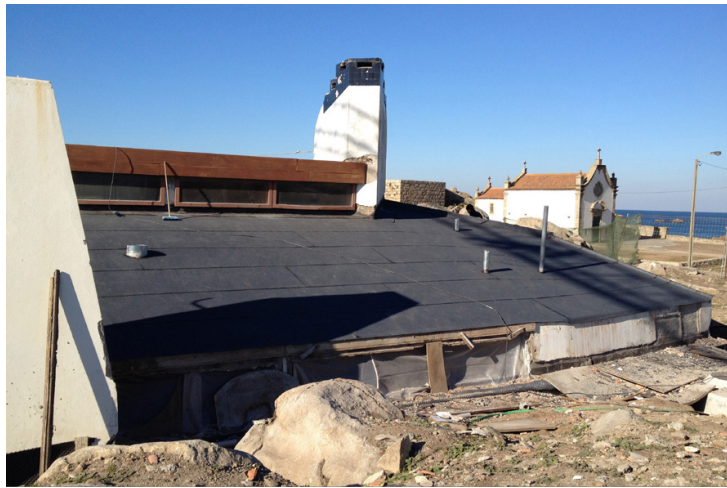
30. Replacement of the roof tiles and waterproofing membranes.
