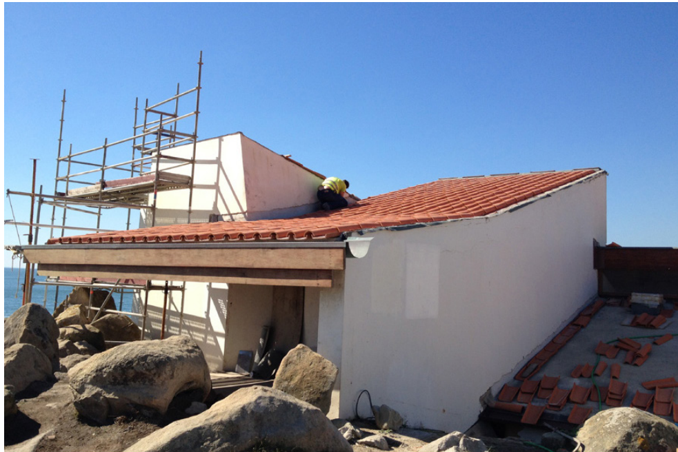
31. Replacement of the roof tiles.
