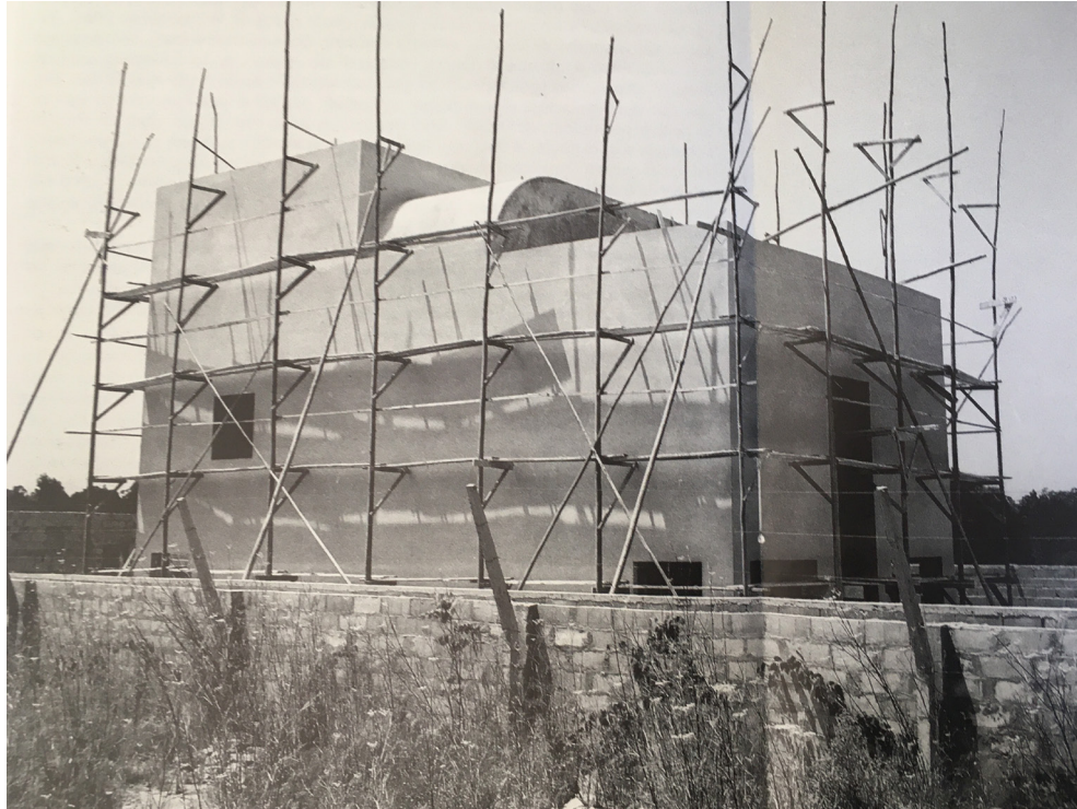
45. Wooden scaffolding used for external plastering.
