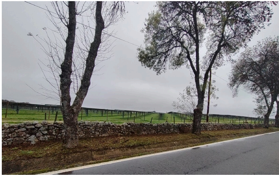
Fig. 3. – View of the existent, Tendeiros, solar plant in Castelo de Vide.
