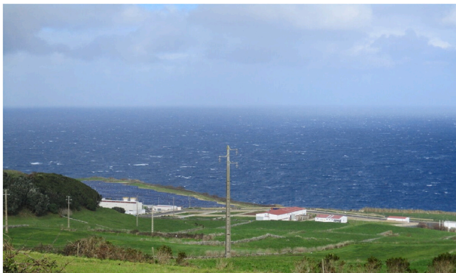
Fig. 2. – View of the solar plant in Graciosa.
