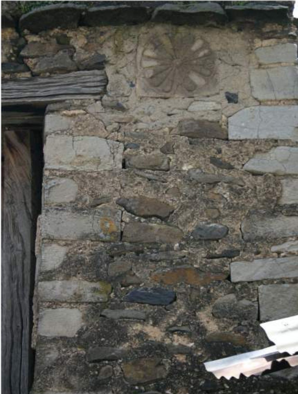
Figure 17 – Inlaid rosette in the upper part and stones cut at the corners of a tower at Täklä Haymanot church of Azezo (photo 2006, Pennecc ©)
