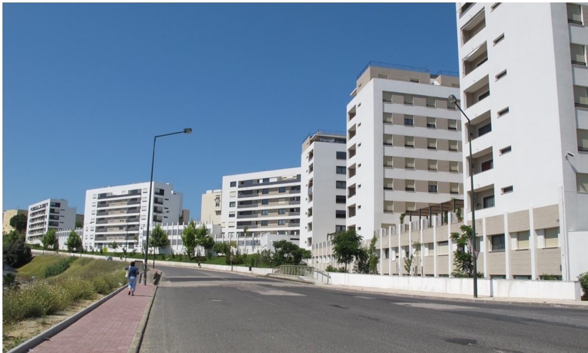
Figure 5 – The “bunker”, Zona J. Source: author.
