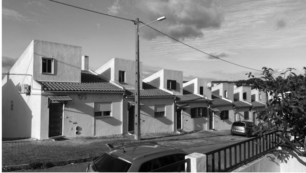
fig. 9 Phase 2 of the Catujal Workers Estate, 2023.
