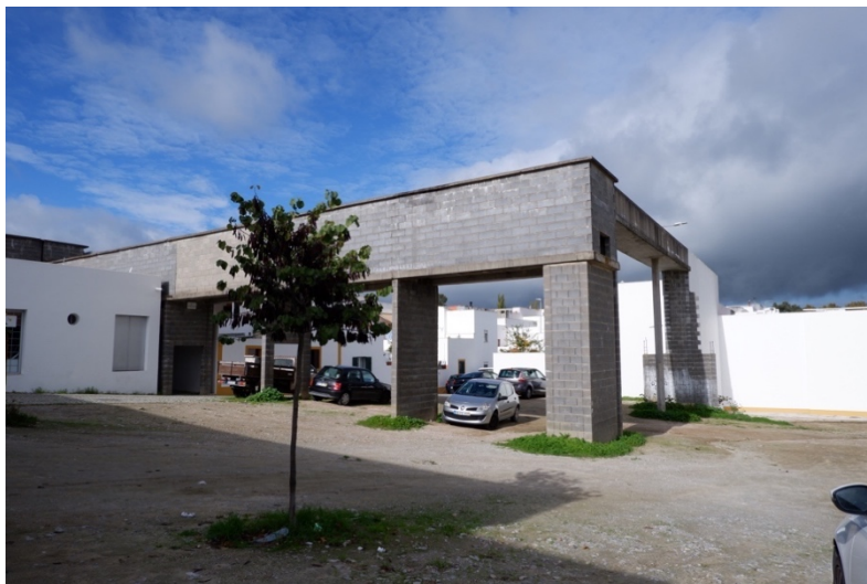
Figure 43. Parking lot in urban void. By author.
