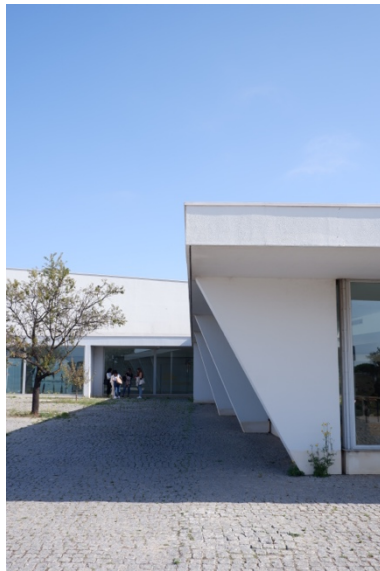
Figure 7. Main Entrance by author.
