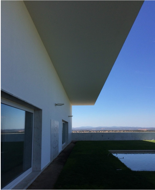
Figure 15. Roof view. by author.
