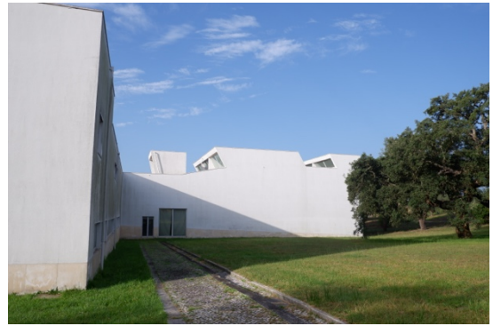
Figure 10. Gym Roof. by author.
