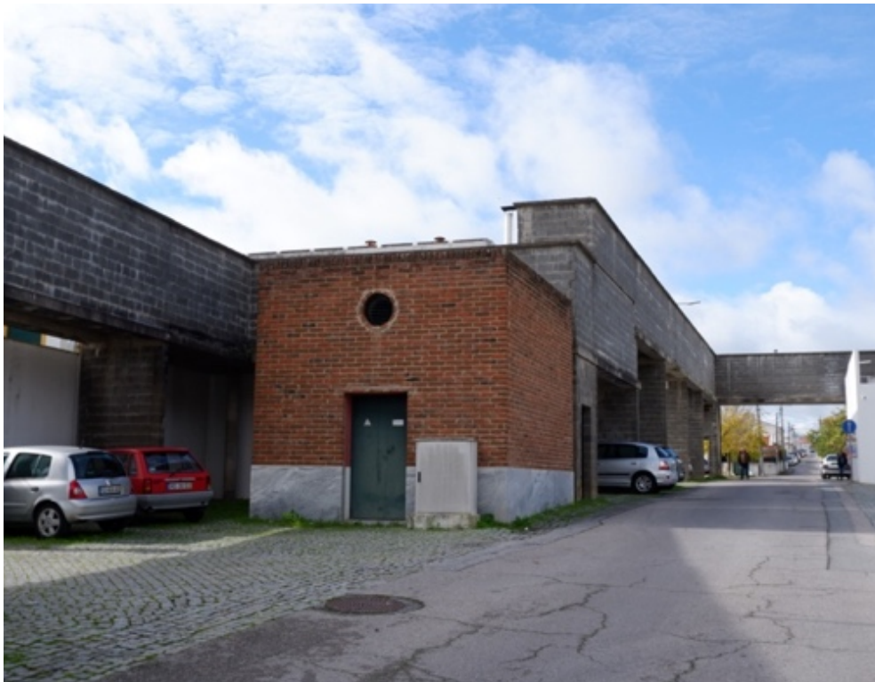
Figure 51. electrical instalations. By author.
