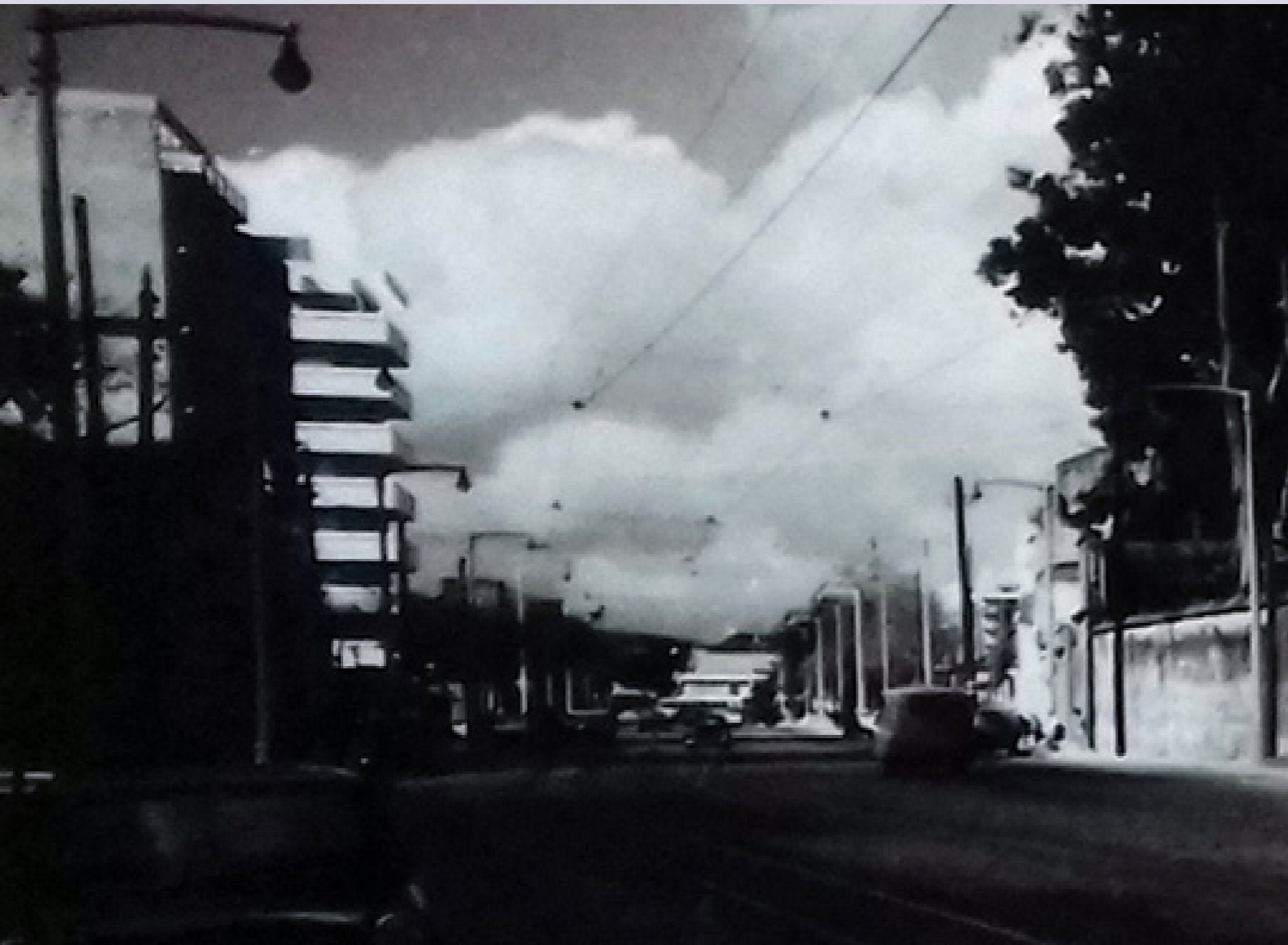
Middle-class building by Fernando Silva in the suburbs of Lisbon, 1968. Street view (© Lisbon city council archives)
