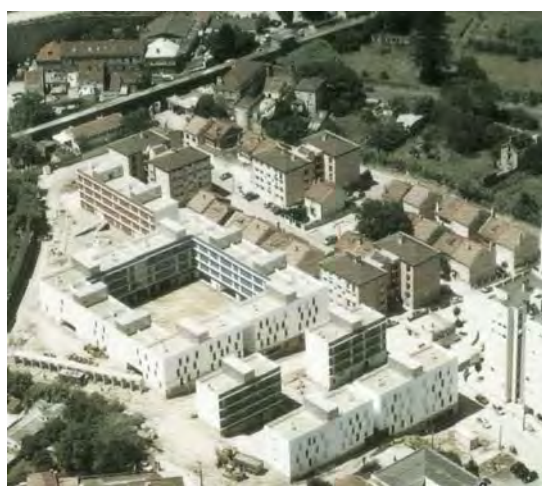
Figure 7. Sargento Abílio Neighborhood during construction. © CML archives
