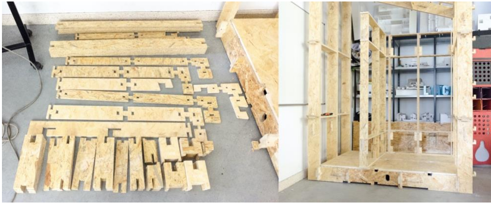
Figure 5-31: (Left) Frame Parts sorted by type before assembly (Right) Assembled frame at Vitruvius FabLab in 2017
