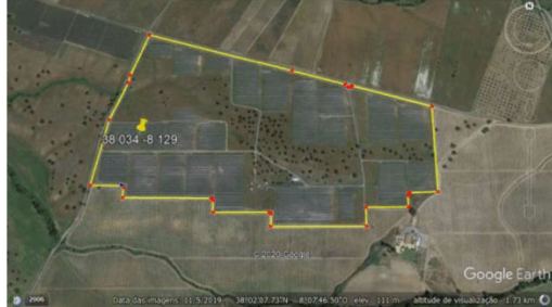
Figure 1: “Ferreira do Alentejo” PV station: installed capacity 12.7 MW_{DC} , total land area 56.5 hectare.
