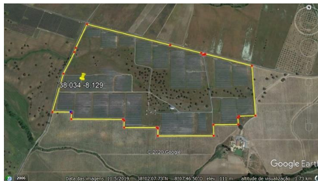
Figure 2.16 – Measuring the “Ferreira do Alentejo” PV power plant (Távora et al., 2020).
