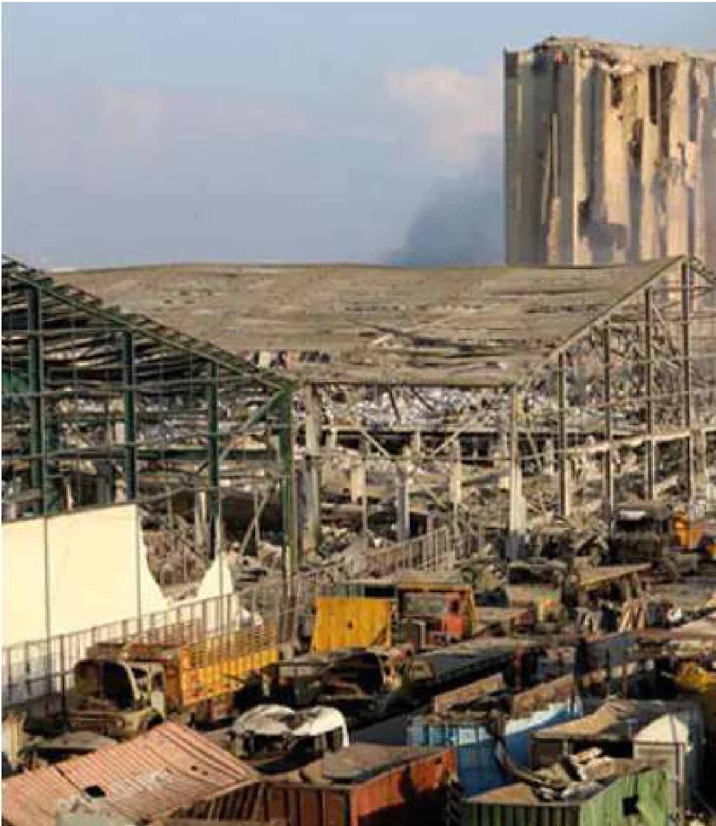
Figure 11: A view shows damages at the site of blast in Beirut's port area
