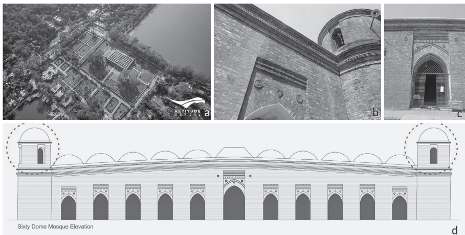
Fig. 4. (a) Site and surroundings of Sixty Dome Mosque (Photo credit: Afzal Nazim), (b) Corner turret and secondary entrance, (c) Main entrance on the East, (d) Elevation showing non-identical design of corner turrets (clockwise).
