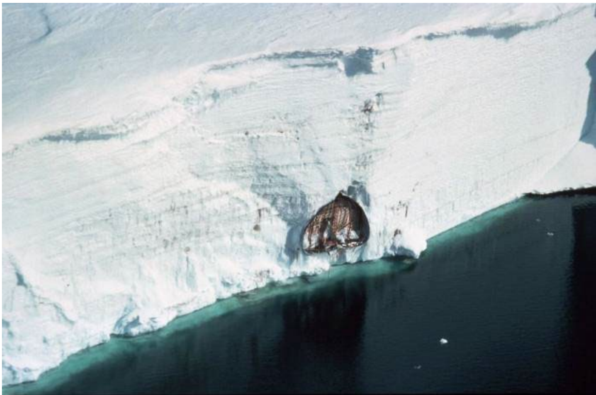
Image 1.16 – Halley III Station, buried and soon to calve off the Brunt Ice Shelf ( N. E. Council, 2013 ).
