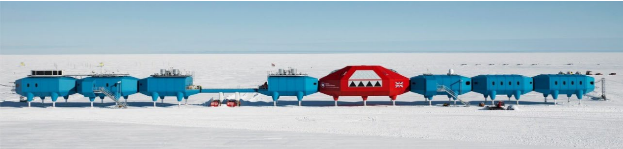
Image 1.20 – Exterior photo of the Halley VI Research Station, with the big red social module in the middle (Hugh Broughton Architects, 2019).
