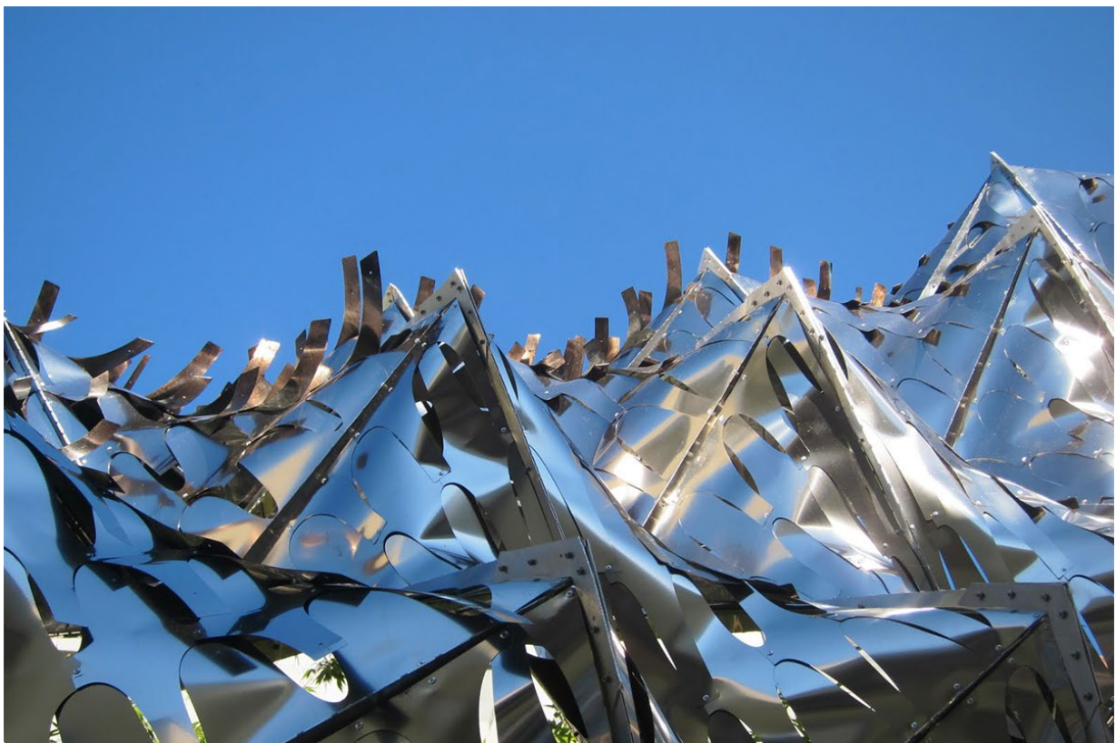
Image 1.12 - Responsive installation "Bloom" by Professor Doris Kim Sung, presented in 2012 at the Materials & Applications gallery in Los Angeles. The façade consists of 14 thousand smart thermobimetal tiles, which curl up when the temperature rises outside or they are hit by sunlight (Sung, 2011).
