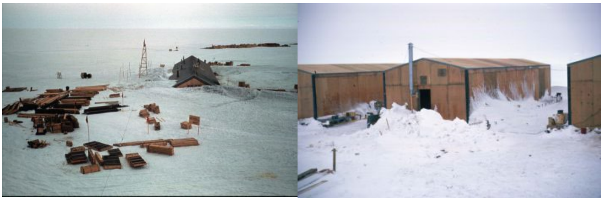
Image 1.17 and 1.18 – Photographs of Halley Station I and II, respectively. Halley Station I was buried under 14 meters of snow, when it was abandoned in 1968, and Halley Station II was only operable for 6 years (1967-1973), as the new steel-reinforced roof was not enough to hold the ice (Nielsen, 2017).
