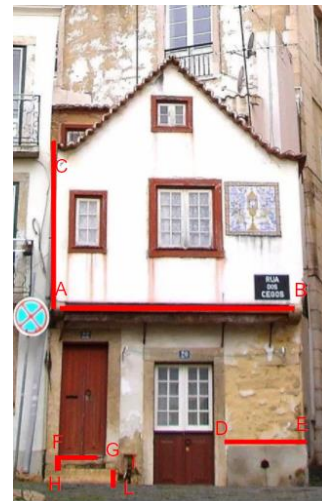
Figure 11. Case study No.1: Measurements from on-site survey used for model scaling the model (DE) and metric comparison.
