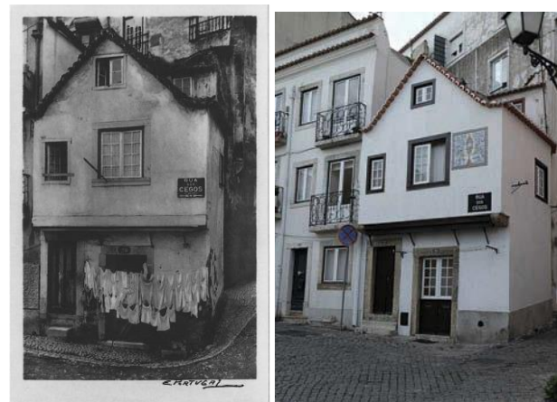
Figure 2. Main façade of case study No.1, Rua dos Cegos no.20, Lisbon: (left) in 1940s (Passos, 1997) vs (right) in 2020s.
