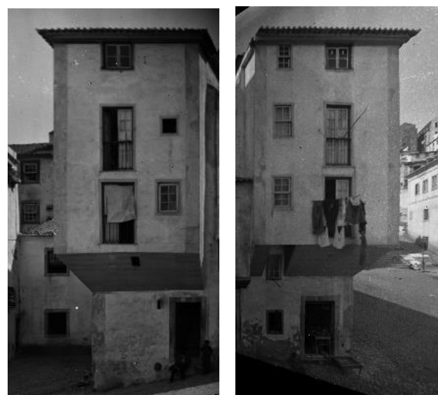
Figure 12. Case study No.2: Rectification of the main building façades of using archival photograph taken by unidentified author (1889-1908).
