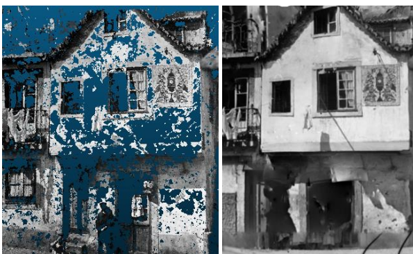
Figure 10. 3D photogrammetric reconstruction of case study No.1, using archival photograph taken by unidentified author (n.d.).
