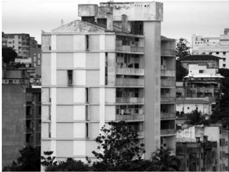
Picture 1. Tonelli , service galleries (arch Pancho Guedes)
