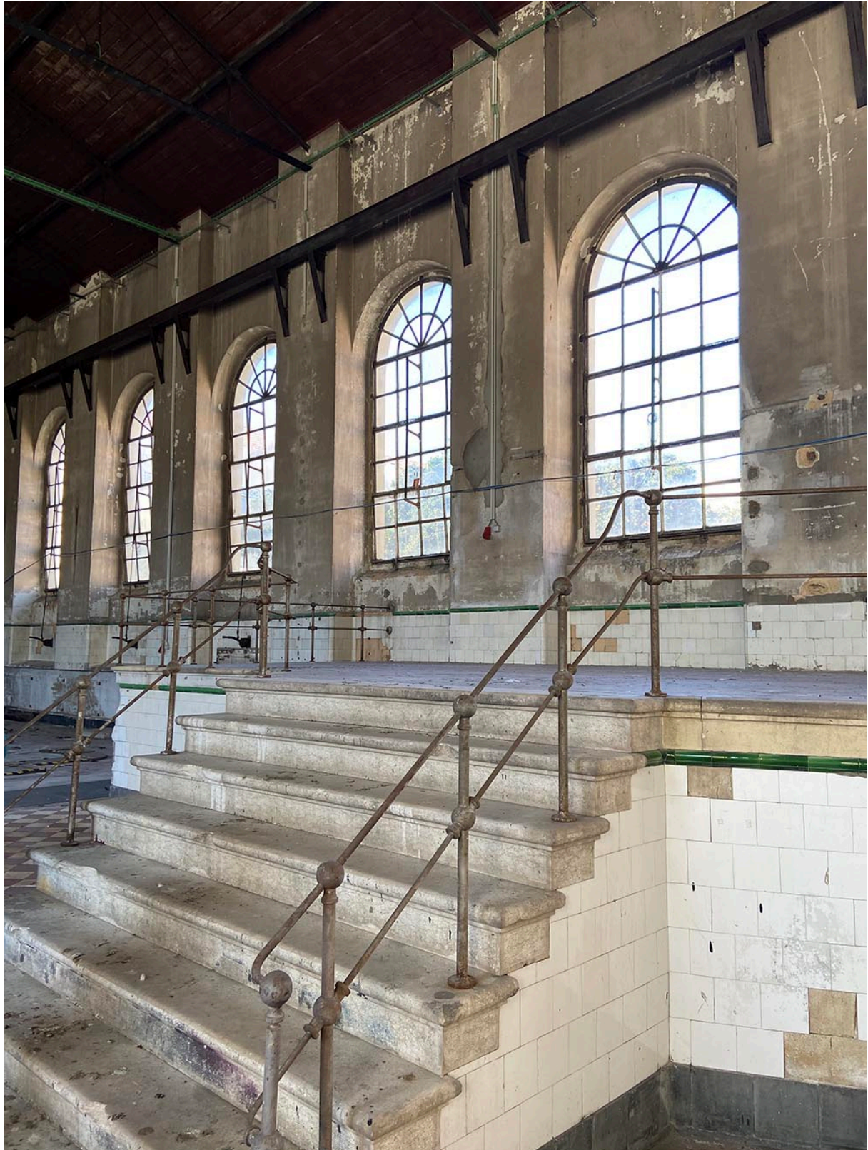
Figura 4.69 – “Central a diesel”.
