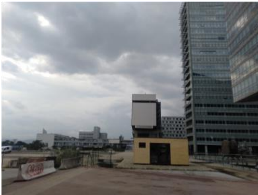
Figure 6. Work in progress
