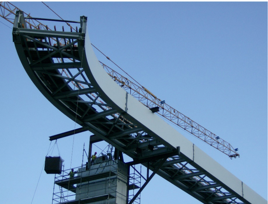
Fig. 5 – Position after the deck lifting, with mounted lateral supporting structure and torsional balancing system.
