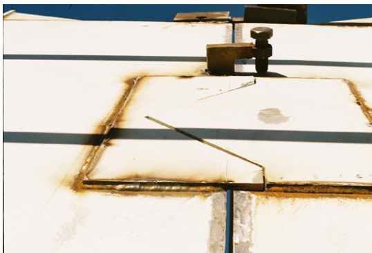
Fig. 11 – Prestressing application and temporary fit.
