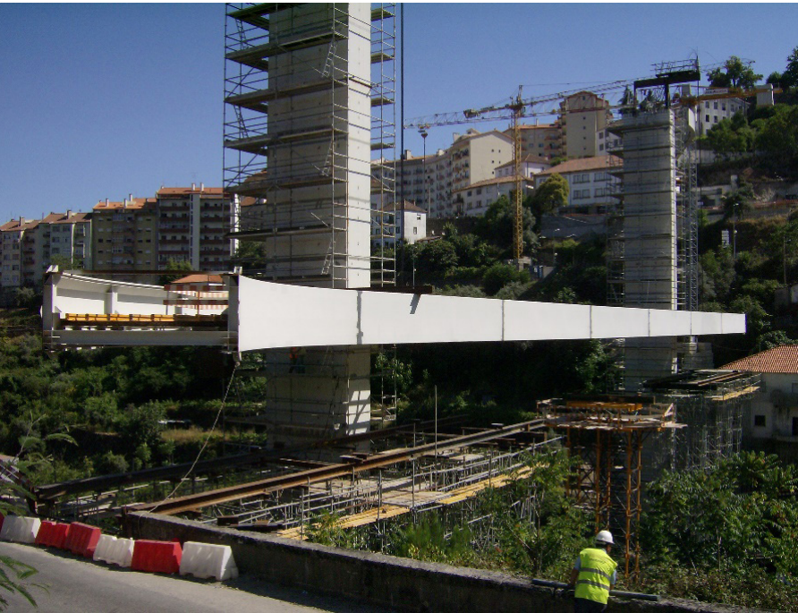
Fig. 4 – Lifting of the central part of the deck suspended on two cables.
