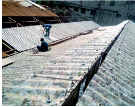
Figura 202 Montagen telhas TuffRoof (Hebel, Wisniewska, & Heisel, 2014)
