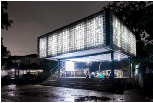
Figura 153 Vista Exterior Bima's Microlibrary (Griffiths, 2016)
