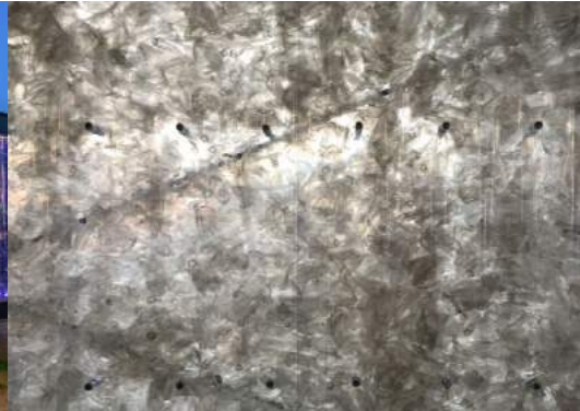
Figura 160 Textura Parede Pet Pavilion (Archdaily, 2014)
