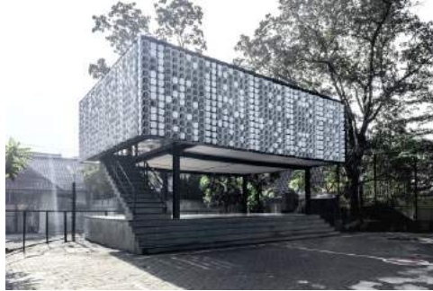
Figura 152 Vista Exterior Bima's Microlibrary (Griffiths, 2016)
