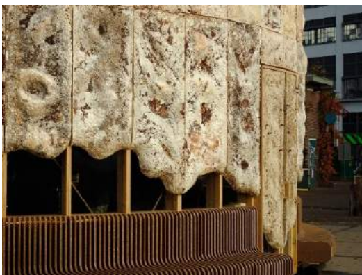
Figura 308 THE GROWING PAVILION (Pownall, 2019)
