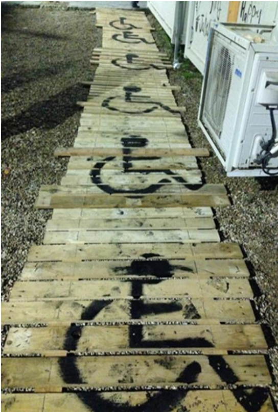
Figure 4.5: Ramp built during the activity Green Street, for an habitant in a wheelchair. (November 2019)
