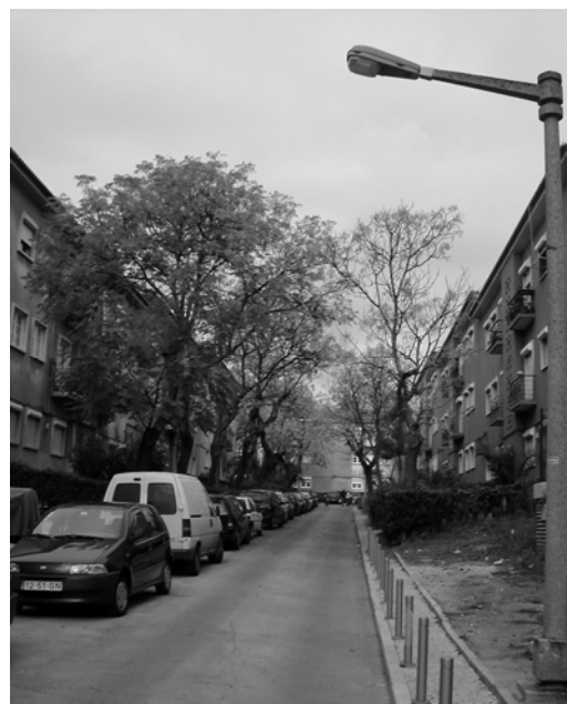
Fig. 2 - Multi-occupancy habitational building in Lisbon, Bairro de Alvalade, decade of 1950.
