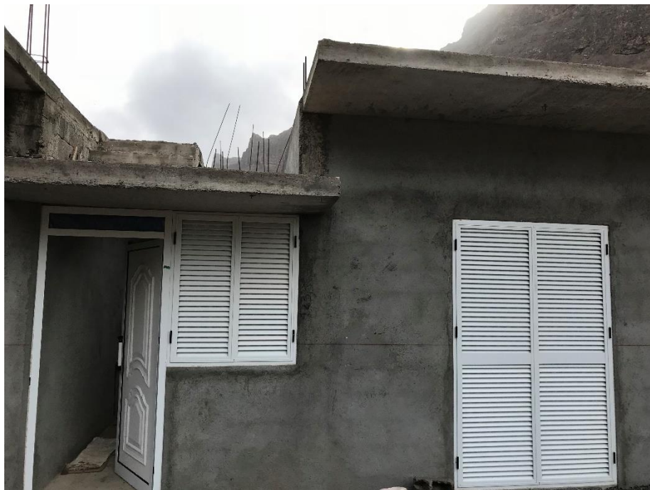
Fig. 4-9 Aspiring modern house in construction, Santiago, 2018.
