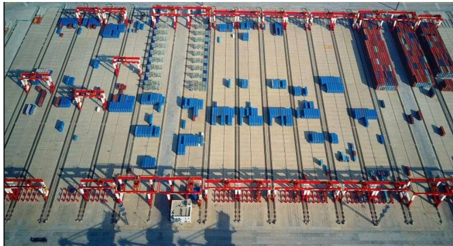
Figure 5.12 - The yard area of the Yangshan port phase4
