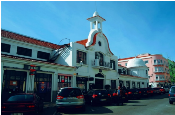
Fig. 6- Eastern façade of the Campo de Ourique Market
