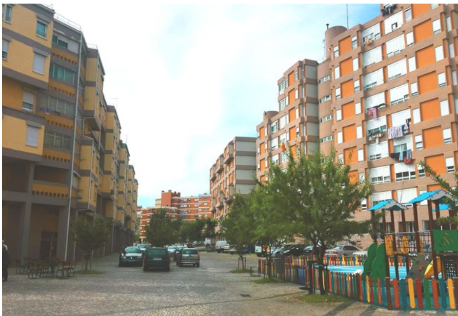
Fig.12 Zone I central strip (Photo: JCB)
