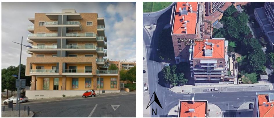
Figure 23 - Kindergarten, the case study building
