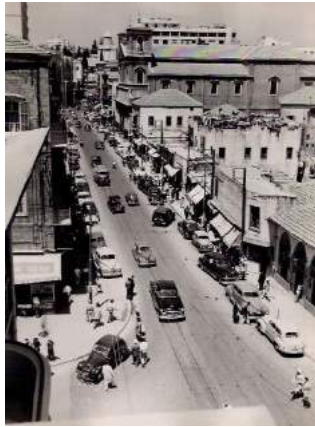
Figure 28: Intersection of Prince Bashir Street and Bchara El Khoury Street - in 60 th .
