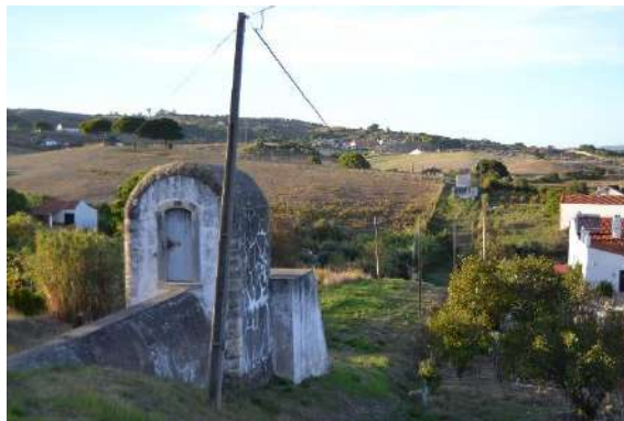
Figure 8 – Alviela Aqueduct in the neighborhood of Quinta da Marmeleira Source: Author.
