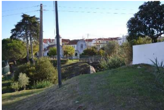
Figure 7 – Alviela Aqueduct in the neighborhood of Paredes. Source: Author.
