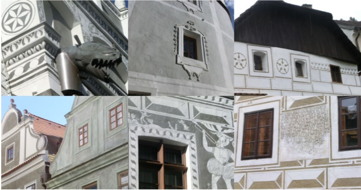
Figure 14.3 Details of the renovated facades of historic centre (author's photos).
