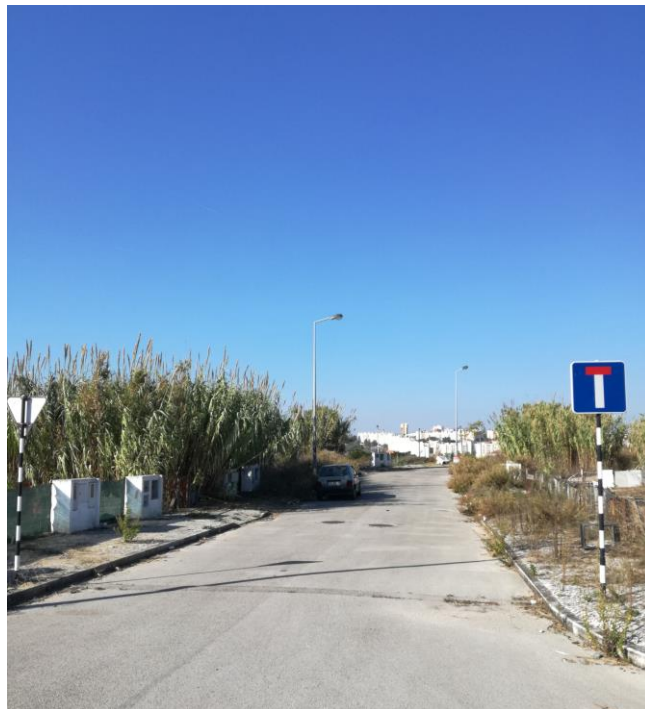
Figure 9 Degradation in an empty allotment operation. From authors, Almada , 2017 (personal collection).
