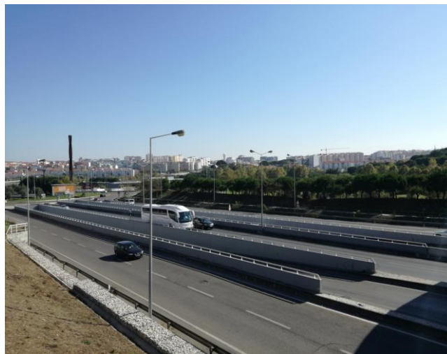
Figure 7 Barrier effect caused by road infrastructure (IC20). From authors, Almada ,2017 (personal collection).
